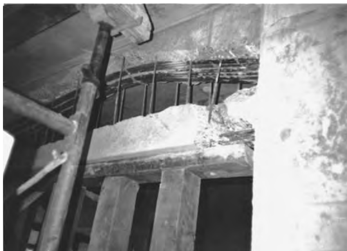
FIGURE 12.22 Misaligned tendon revealed by destructive testing.
