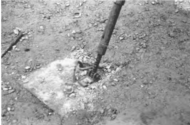
FIGURE 7.20 Formwork brace anchored to buried concrete mass.
