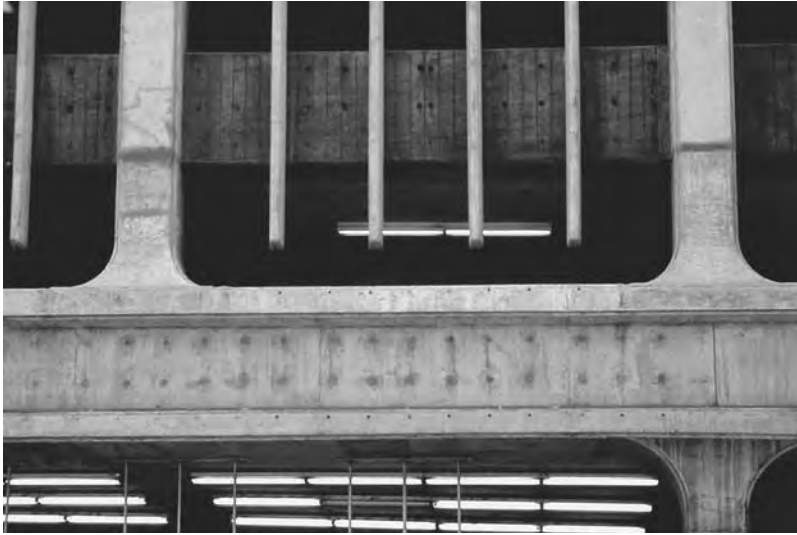
FIGURE 30.18 Dark leakage areas around form tie holes where moisture has migrated, resulting in localized concrete with a lower w/c ratio.
