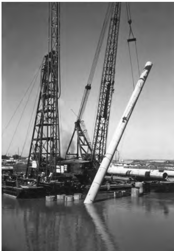
FIGURE 11.42 Prestressed concrete cylinder pile for pier of Napa River Bridge in California. (From Gerwick, B.C., Jr., Construction of Prestressed Concrete Structures , John Wiley & Sons, New York, 1996. With permission.)
