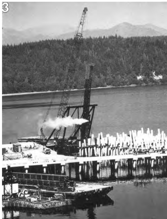
FIGURE 11.51 Driving long prestressed concrete piling for major naval facility in Puget Sound, Washington.
