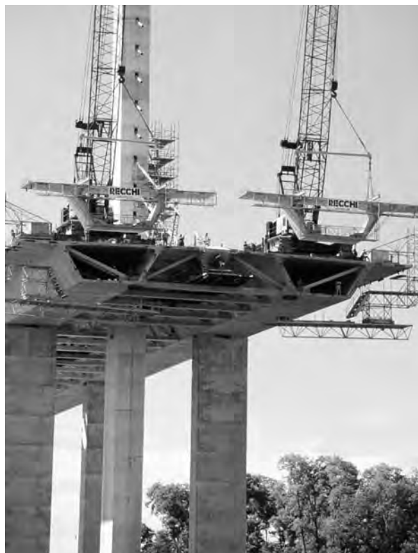
FIGURE 29.16 Precast delta frames between the parallel box girders transfer forces from the superstructure to the cable stays.
