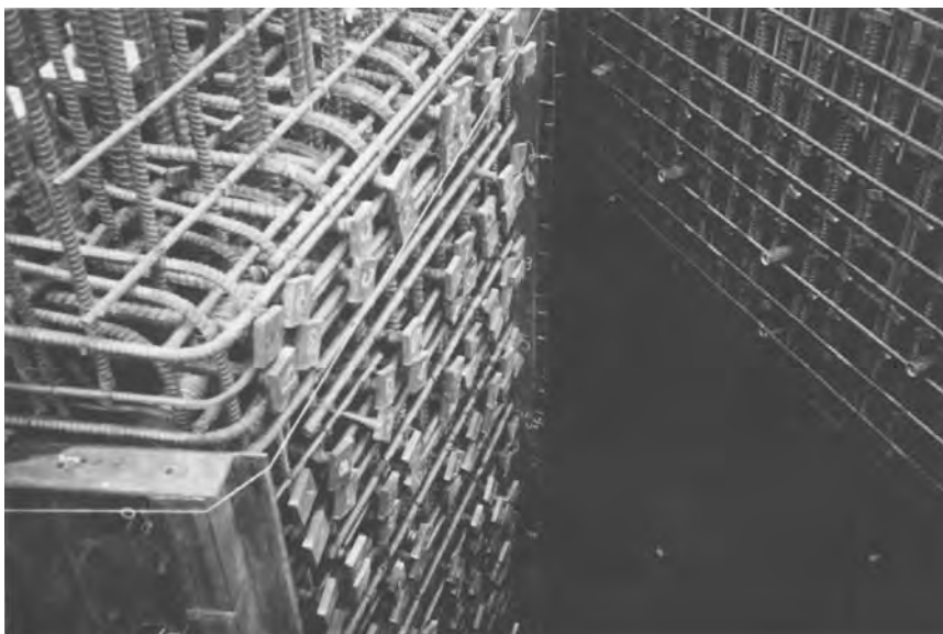
FIGURE 11.5 Mechanically headed bars used to replace conventional closed stirrups.
