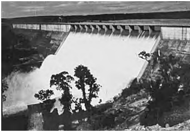
FIGURE 20.3 Urugua-I Dam in Argentina, which used 105 lb of cement per cubic yard (no ash). (Photograph courtesy of Ernest K. Schrader.)
