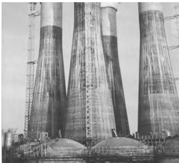
FIGURE 11.2 Statfjord B offshore platform with prestressed concrete shafts. (From Gerwick, B.C., Jr., Construction of Prestressed Concrete Structures , John Wiley & Sons, New York, 1996. With permission.)
