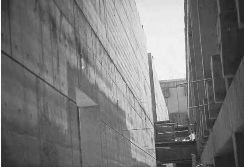
FIGURE 30.3 Waviness in the concrete surface due to lack of form rigidity during concrete consolidation.
