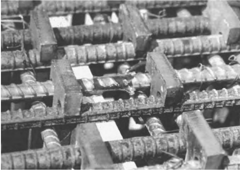
FIGURE 11.4 T-headed bars lock against reinforcing steel to provide high shear capacity and confinement.
