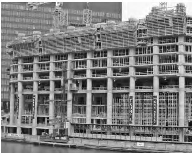
FIGURE 19.30 Crane-independent self-climbing forming system (Trump Tower, Chicago).
