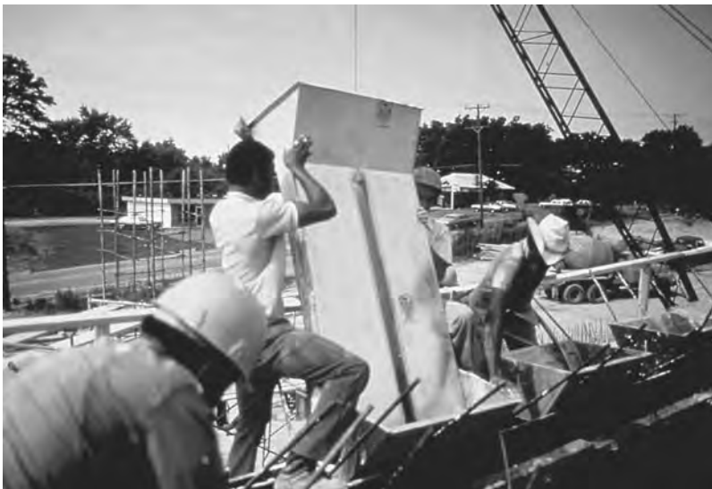
FIGURE 30.32 Tremie being placed in position for use.
