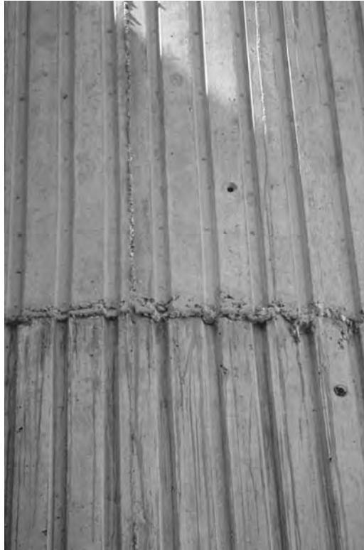
FIGURE 30.17 Spill or overpour at construction joint during placement and consolidation. Tying the form into the previous concrete placement and installing a compressible gasket in the reveal would have prevented this leakage.
