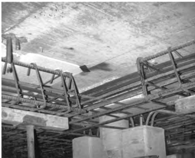
FIGURE 12.34 Tendons installed within a reinforcing cage.
