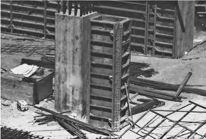
FIGURE 7.11 Modular steel form for rectangular columns.
