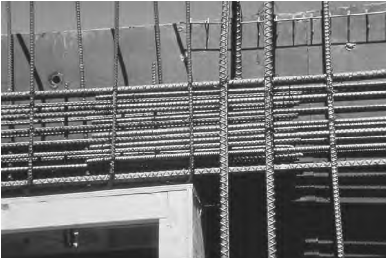
FIGURE 30.22 Lapping of bars all occurring at one location causing congestion that can lead to honeycombing.
