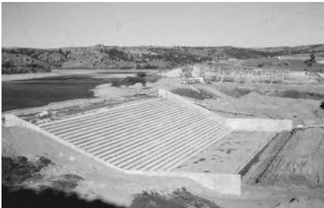
FIGURE 20.10 RCC used to provide a buttress and overtopping spillway for the Tongue River embankment dam in Montana. The mix primarily used 150 lb of cement (no ash) with surface layers of the stilling basin having higher cement content.
