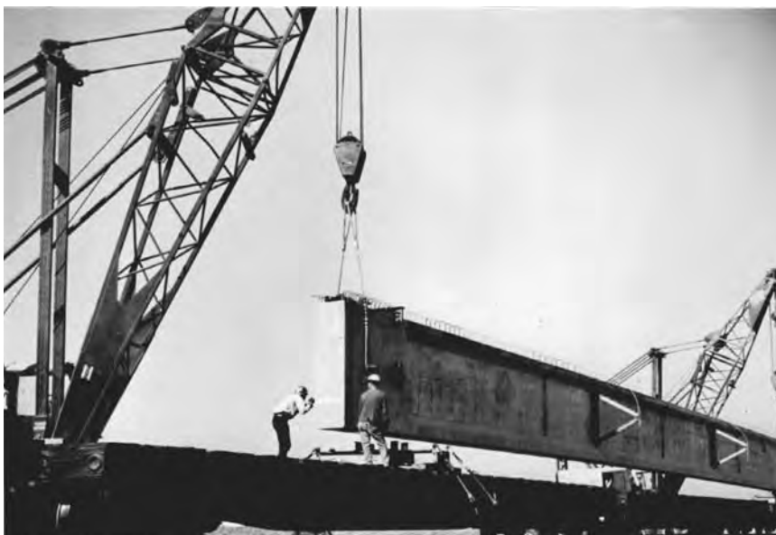
FIGURE 11.13 Prestressed lightweight concrete girder being prepared for shipment by rail. (From Gerwick, B.C., Jr., Construction of Prestressed Concrete Structures , John Wiley & Sons, New York, 1996. With permission.)
