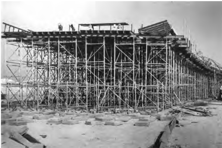
FIGURE 7.2 Formwork elements must support many heavy loads.
