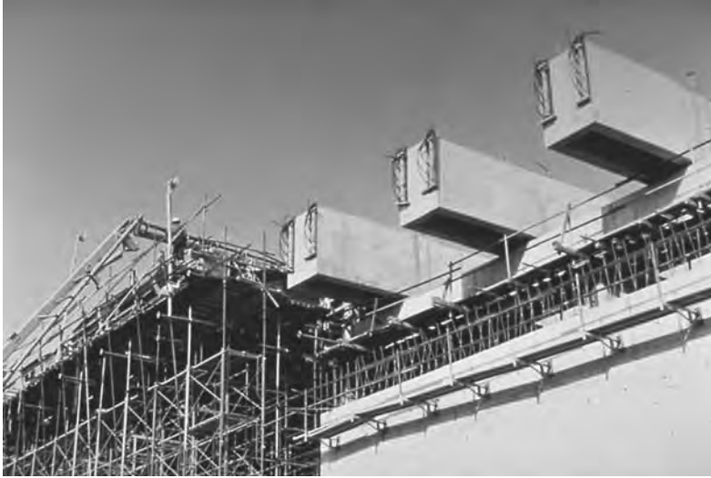
FIGURE 30.28 After cutting, the strands were grouted in the sheathing, and the recess was filled with architectural concrete patch mix, covered with wet burlap, and protected with a wood cover.
