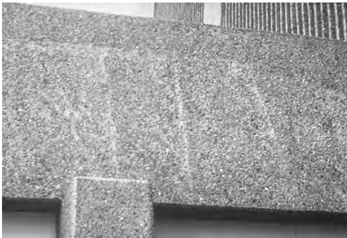
FIGURE 30.36 Grout lines on exposed face of architectural concrete due to an internal vibrator touching the side of the form during concrete consolidation.
