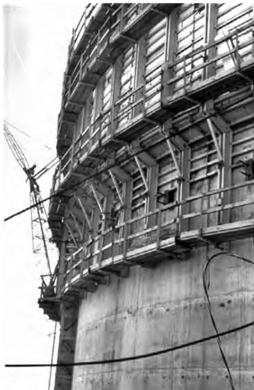
FIGURE 7.6 Custom-made steel form with integrated access platforms.
