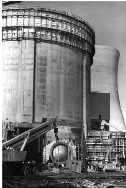
FIGURE 7.3 Large and complex placements require substantial formwork.
