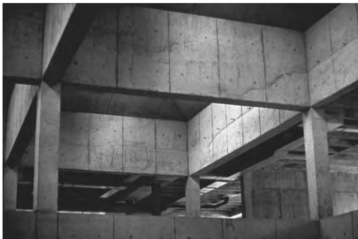
FIGURE 30.7 Pour lines on interior beams where the concrete was placed during hot weather. Higher dosages of admixtures could have been used to minimize the possibility of early set leading to pour lines.
