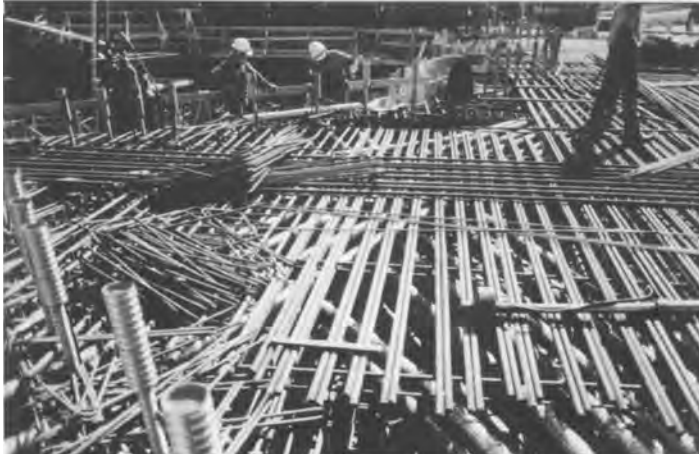
FIGURE 11.10 Congestion of conventional reinforcement and multi-axial prestressing ducts creates problems for concrete placement. (From Gerwick, B.C., Jr., Construction of Prestressed Concrete Structures , John Wiley & Sons, New York, 1996. With permission.)
