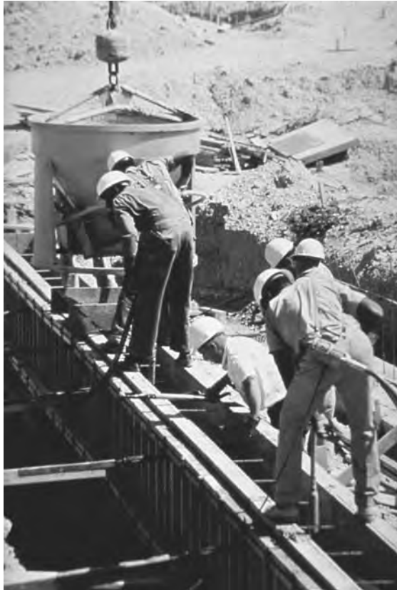
FIGURE 30.35 First operator is vibrating concrete at point of deposit; second operator is blending concrete to eliminate lift lines and minimize bug holes.
