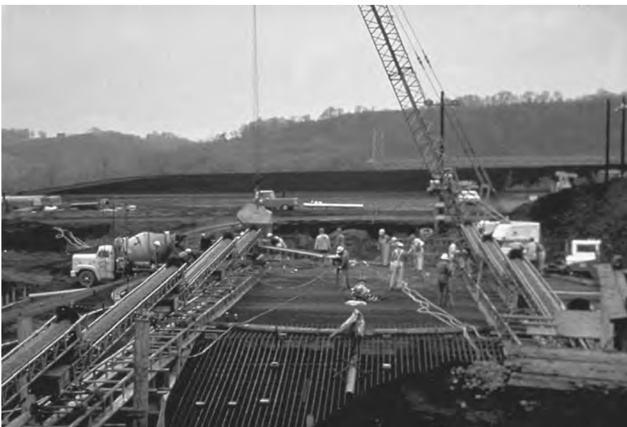
FIGURE 30.30 Conveyors in use at construction site.
