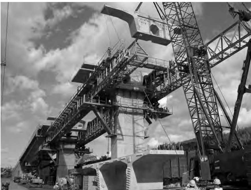
FIGURE 29.14 Span-by-span erection of the approach spans expedited completion of New Jersey’s Victory Bridge.
