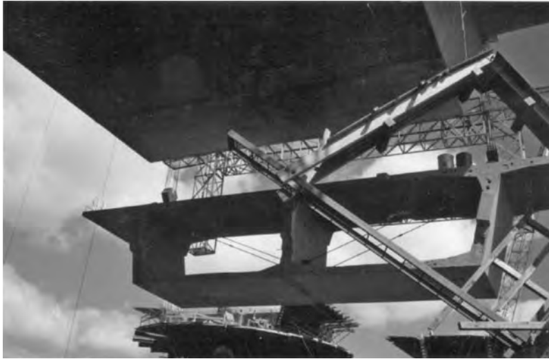
FIGURE 11.37 Erecting precast match-cast segment in cantilever construction.
