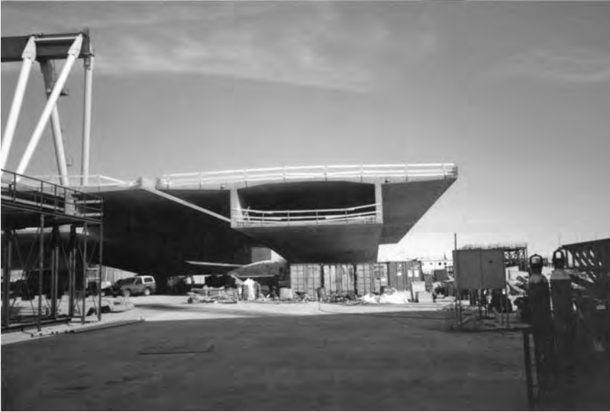
FIGURE 11.38 Full-width, full-length bridge span for the Great Belt Western Bridge in Denmark is prefabricated on land.
