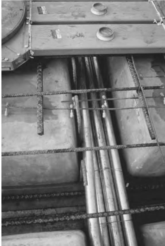
FIGURE 30.19 Electrical conduit blocking access for placement and consolidation of concrete.
