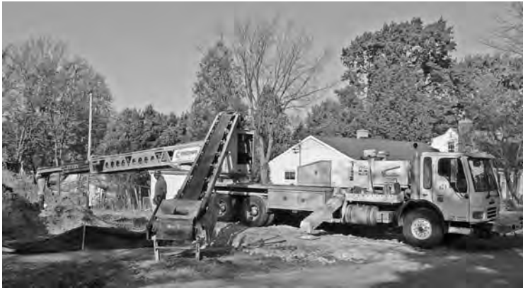
FIGURE 19.26 Truck-mounted telescopic belt conveyor.
