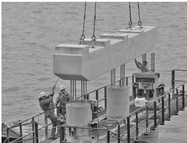
FIGURE 33.17 Precast concrete pier bent. (Figure courtesy of the Texas Department of Transportation, Dallas.)
