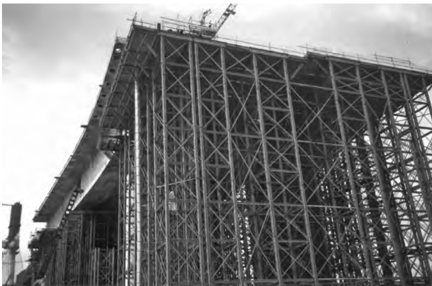
FIGURE 11.32 Structural steel falsework supports high-level cast-in-place post-tensioned bridge (Ma Wan Viaduct, Hong Kong).
