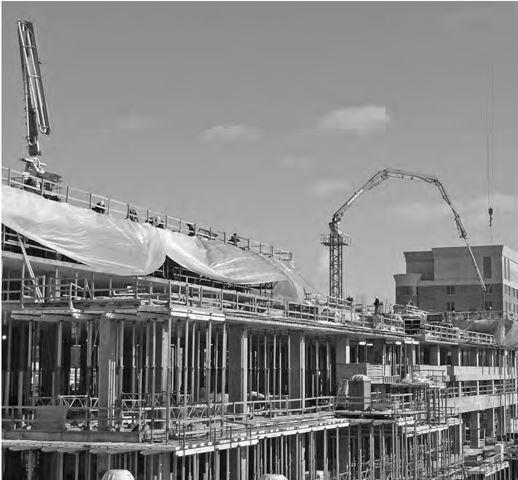
FIGURE 19.7 Climbing placing booms.
