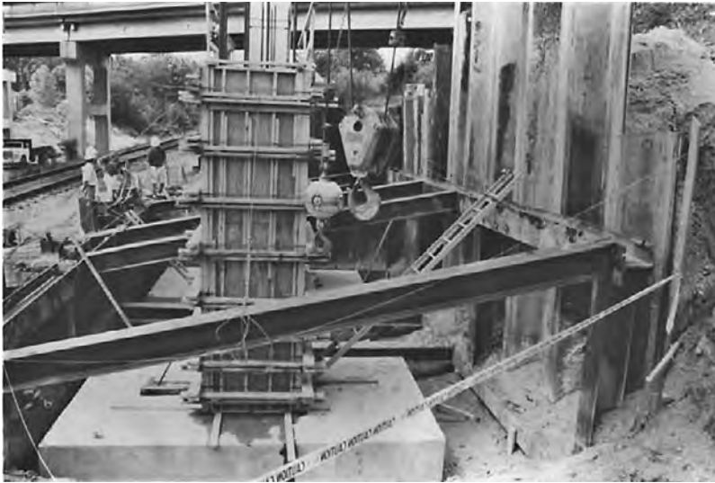
FIGURE 7.5 Wood column form.
