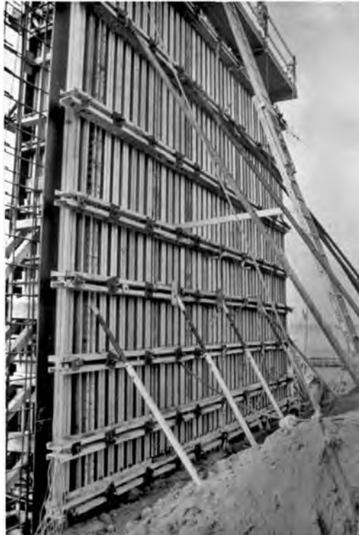
FIGURE 7.28 Tall wall form with internal pressures resisted by ties and wind resisted by external braces.
