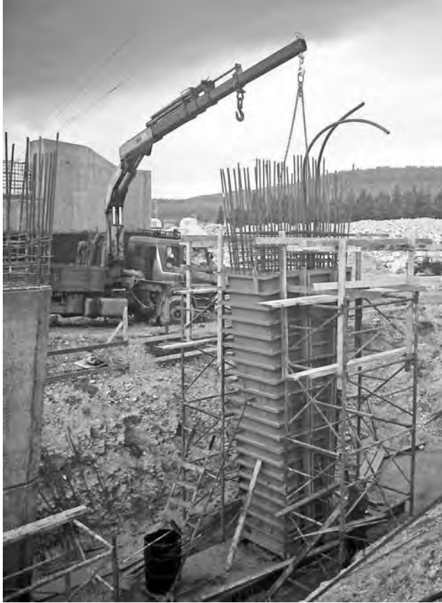
FIGURE 19.25 Knuckle-boom truck loader in form-assembly work.
