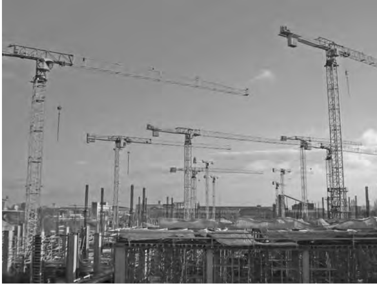
FIGURE 19.13 A cluster of flat-top tower cranes on a commercial building project in Budapest, Hungary. The photograph was taken in January 2007, when the site was inoperative, as is apparent from the weathervaning cranes. (Photograph courtesy Meir Simcha, Israel.)
