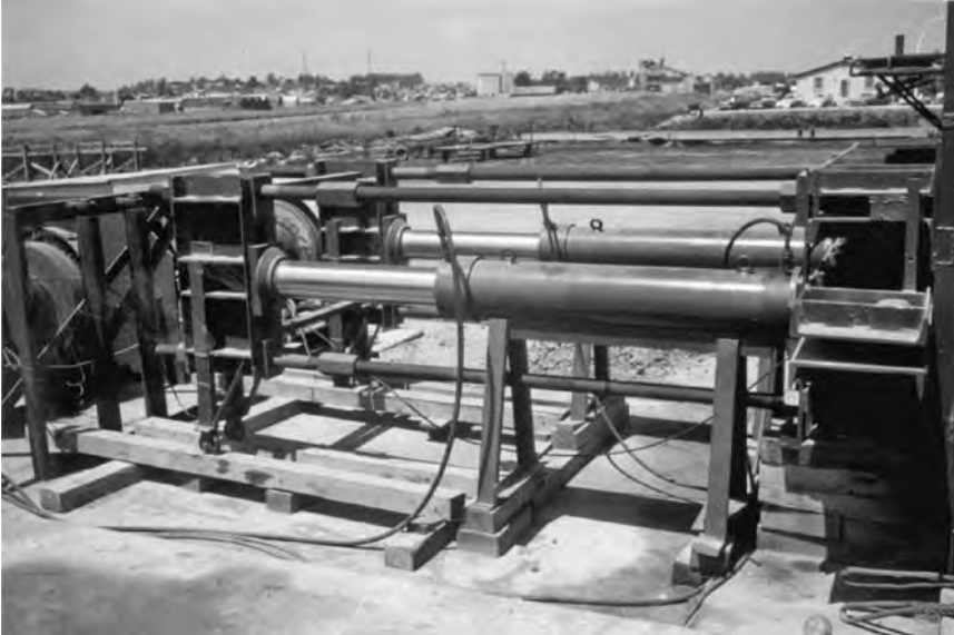
FIGURE 11.21 Fully extended jacks impart prestress to pretensioning strands. (From Gerwick, B.C., Jr., Construction of Prestressed Concrete Structures , John Wiley & Sons, New York, 1996. With permission.)
