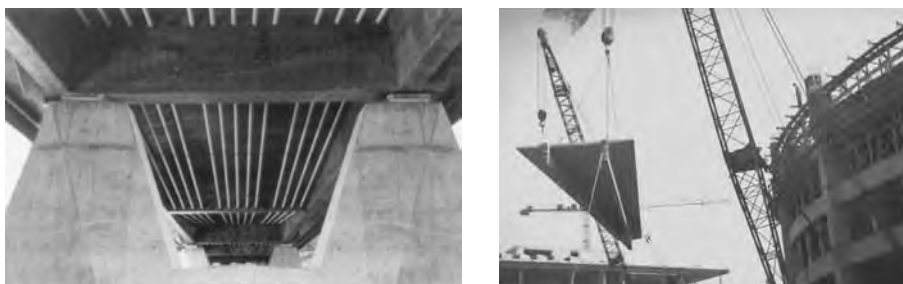
VSL External Post-Tensioning System Components
