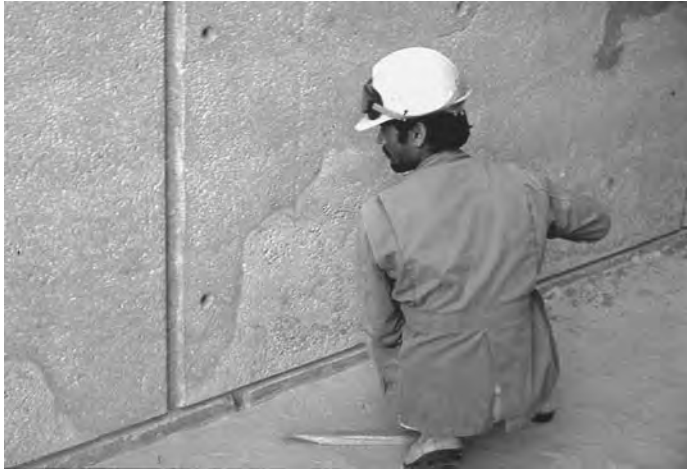
FIGURE 30.34 Adjacent concrete walls from two separate days' placement showing the impact of pumping concrete directly without wasting first 1/4 yd 3 (0.2 m 3 ) to coat the pump and hoses.
