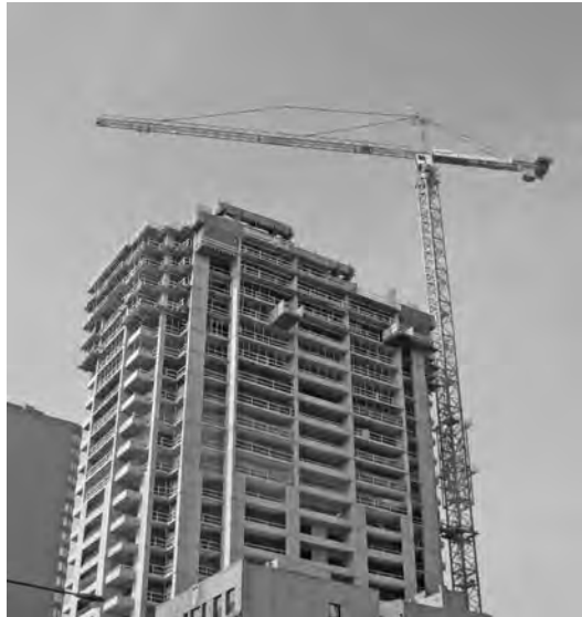
FIGURE 19.9 Top-slewing saddle-jib tower crane.
