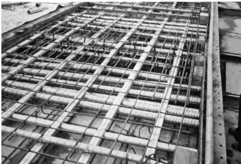
FIGURE 11.9 Both longitudinal and transverse ducts in place to receive tendons after concrete has been placed and cured.
