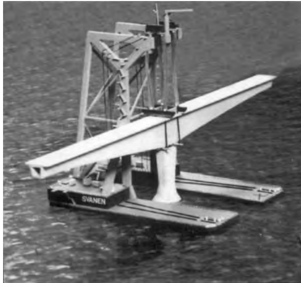
FIGURE 11.39 Erecting one of the 124 spans of the Great Belt Western Bridge in Denmark; each is 100 m long and weighs 7000 t.
