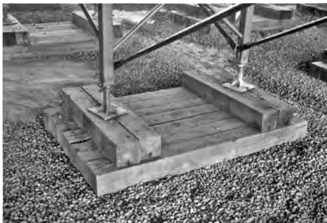
FIGURE 7.36 Wood timber grillage mudsill.
