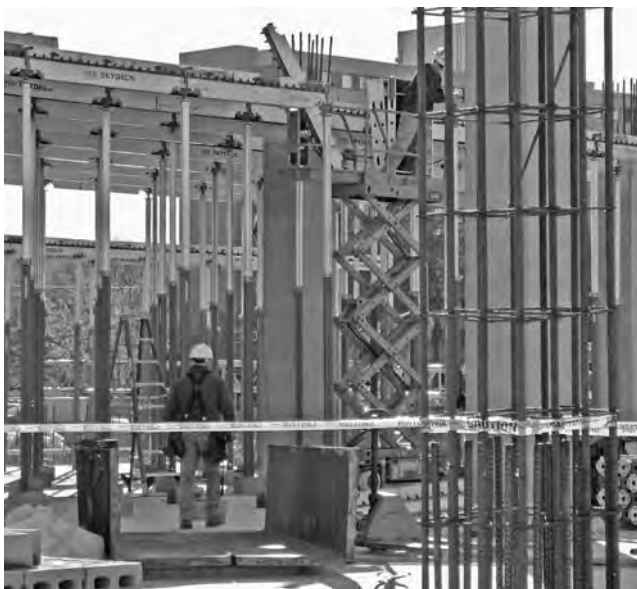
FIGURE 19.28 Scissor lift in slab deck formwork.
