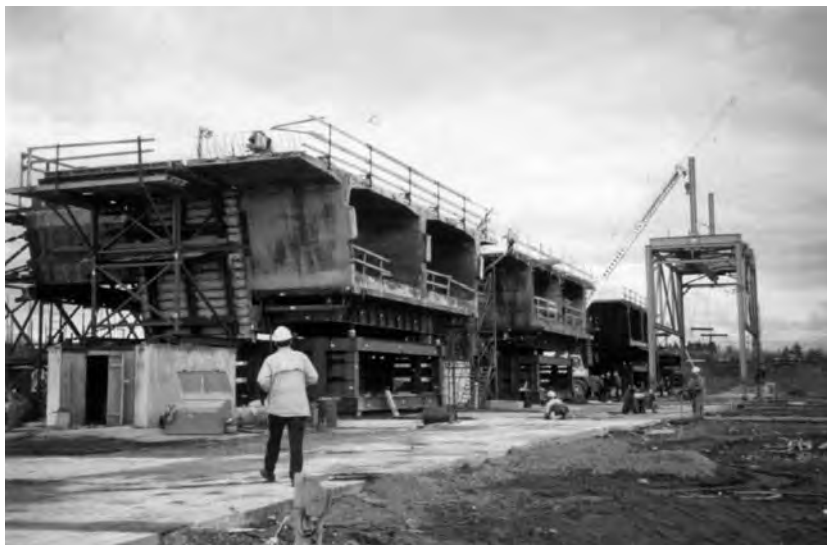
FIGURE 11.34 Precast concrete segments are match-cast in elevated cells to facilitate their alignment and movement.
