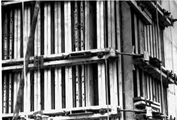
FIGURE 7.35 Connections at corners, braces, and bulkheads require specific design.
