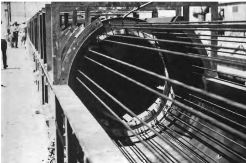
FIGURE 11.45 Closing up forms during manufacture of pretensioned cylinder piles.
