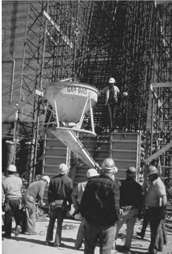
FIGURE 30.29 Steep-sided bucket with easily movable chute to aid in placement of concrete.
