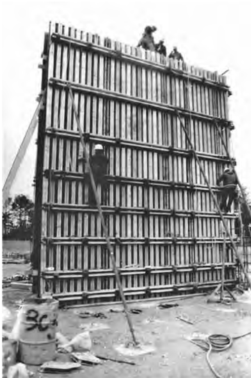
FIGURE 7.25 Preengineered wall form system.
