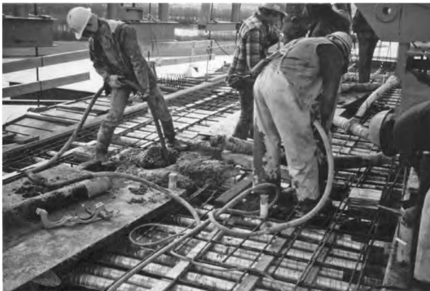
FIGURE 11.11 Vibrating concrete in order to ensure thorough consolidation below ducts. (From Gerwick, B.C., Jr., Construction of Prestressed Concrete Structures , John Wiley & Sons, New York, 1996. With permission.)
