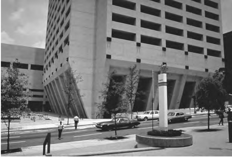
FIGURE 30.10 Heavy jackhammer surface on Southern Bell Tower in Atlanta, Georgia; architect, Skidmore, Owings, and Merrill, Chicago.
