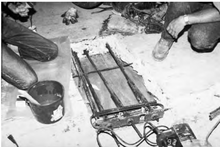
FIGURE 16.14 New anchorages and bursting steel.
