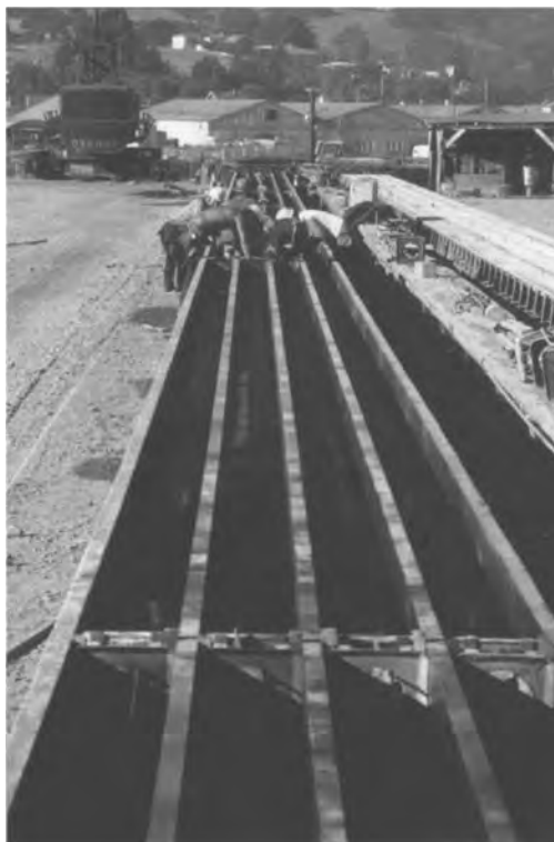
FIGURE 11.20 Stretching strands down pretensioning bed.
