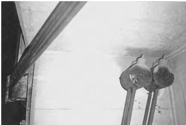
FIGURE 12.26 Alternative connection of external unbonded tendons.
