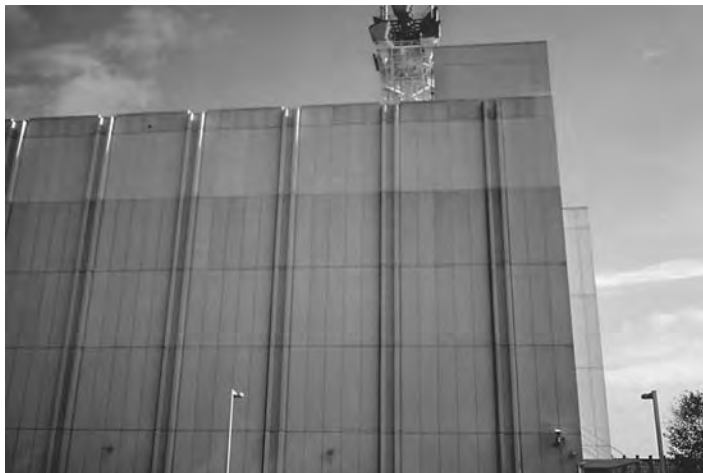
FIGURE 30.8 Precast addition over 15 years later using the same cement, aggregates, and mix design.
