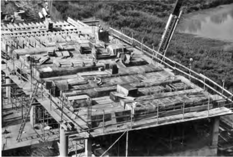
FIGURE 7.22 Guardrails and rated, well-maintained access ladders are components of a safety system.
