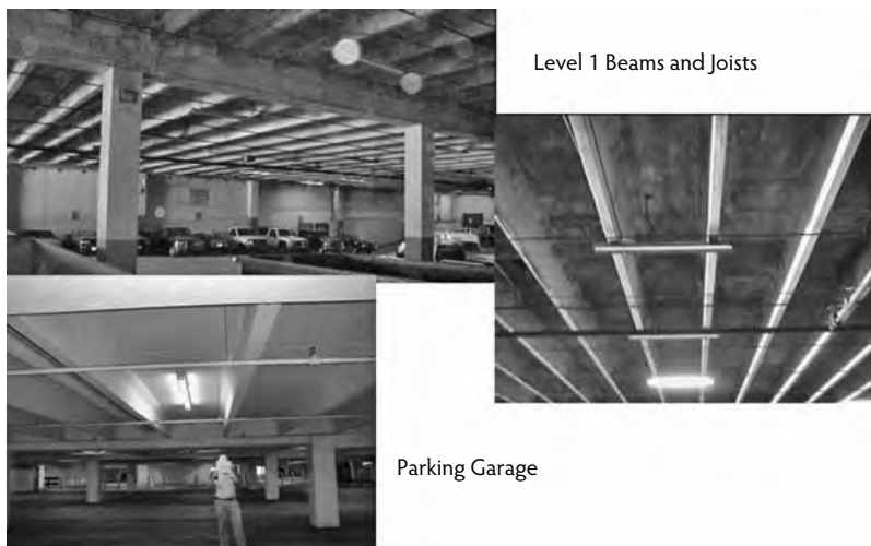
FIGURE 22.19 Upgrade of telecom building using hybrid GFRP-reinforced concrete in beams and joists. (From Nawy, E.G., Concrete: The Sustainable Infrastructure Material for the 21st Century , Circular E-C103, Transportation Research Board, Washington, D.C., 2006, pp. 1–24. Courtesy of Dr. A. Nanni.)
