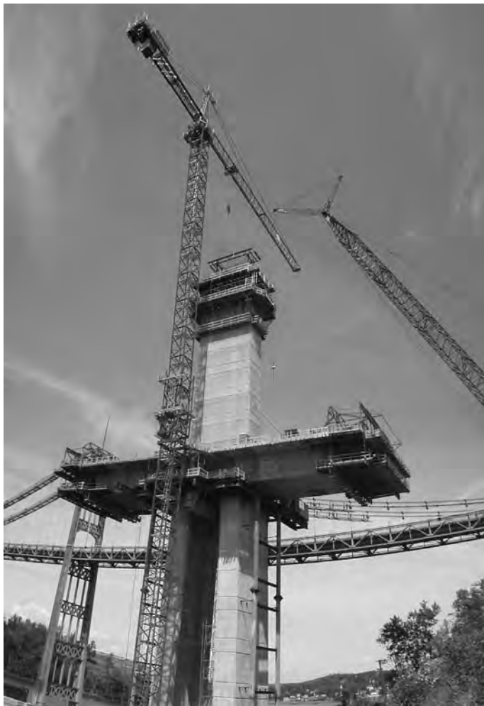
FIGURE 29.17 Form travelers on the cantilever tips were used to cast the superstructure in place for Maine's Penobscot Narrows Bridge and Observatory.
