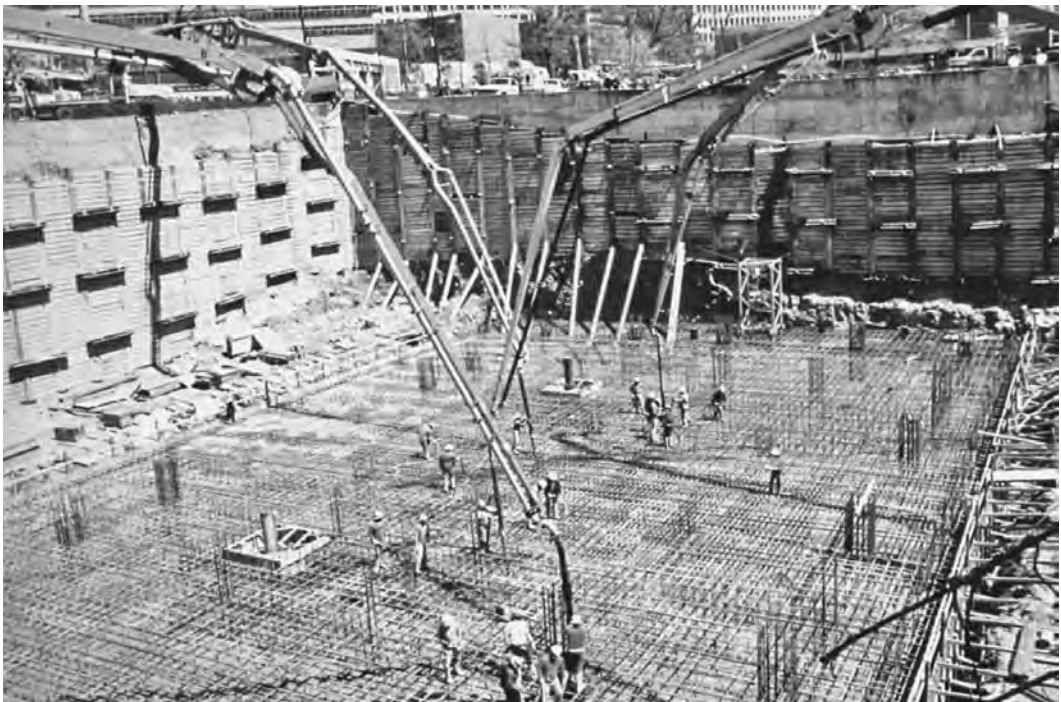
Foundation preparation for high-rise building. (Photograph courtesy of Portland Cement Association, Skokie, IL.)
