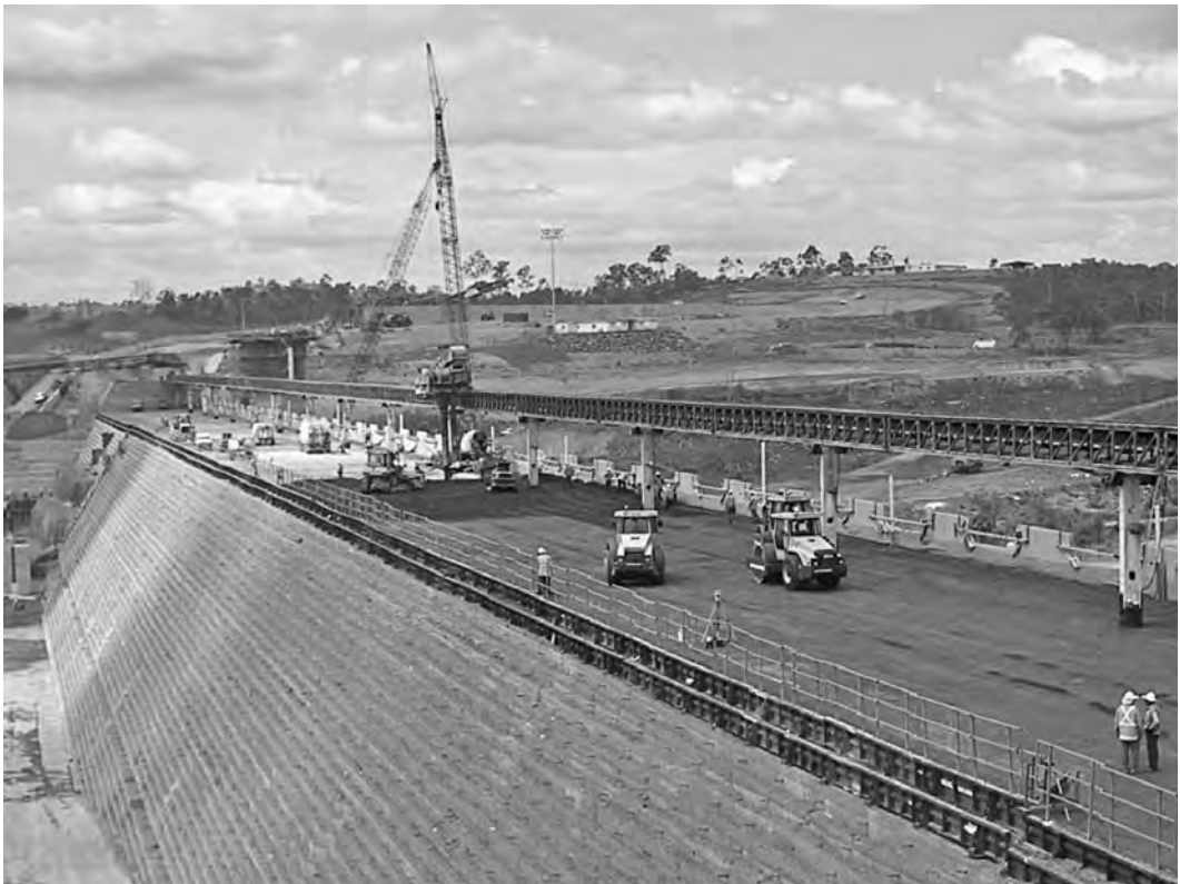
Placing RCC at 500 cu yd/hr, Paradise (Burnett River) Dam in Australia. (Photograph courtesy of Ernest K. Schrader.)
