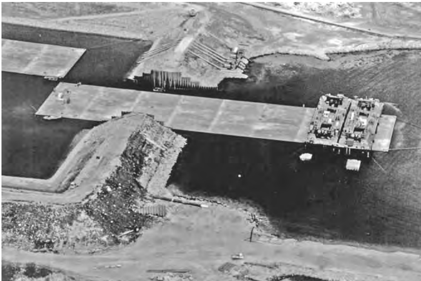
FIGURE 11.55 Temporary post-tensioned segment of the Oresund Tunnel exiting assembly basin. (Photograph courtesy of Oresundbro Konsortiet, Copenhagen, Denmark.)
