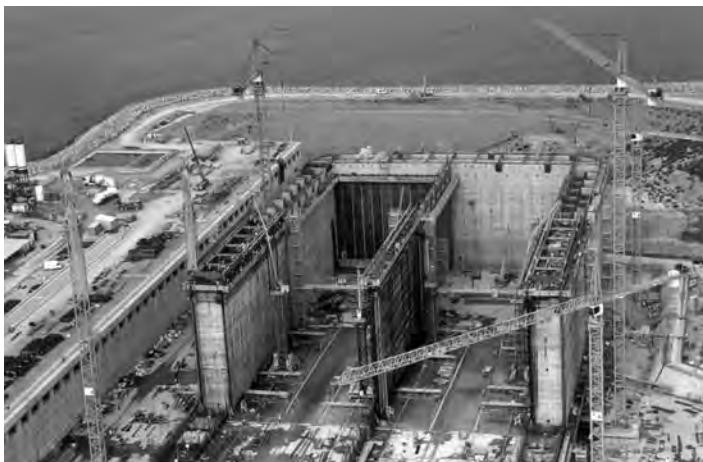
FIGURE 13.8 Dry-dock construction of the reinforced concrete Isola di Porto Levante LNG terminal. (Photograph courtesy of Aker Kvaerner, Lysaker, Norway.)
