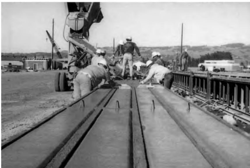
FIGURE 11.22 Concreting and finishing operations.
