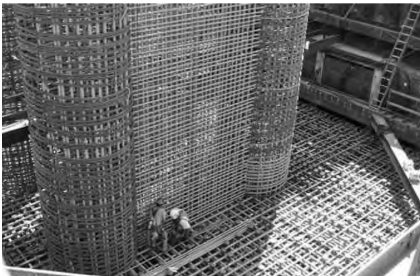
FIGURE 15.13 Overview of footing and pier prior to footing placement. (From Gajda, J., Concrete Technol. Today , 24(3), 34–37, 2003.)
