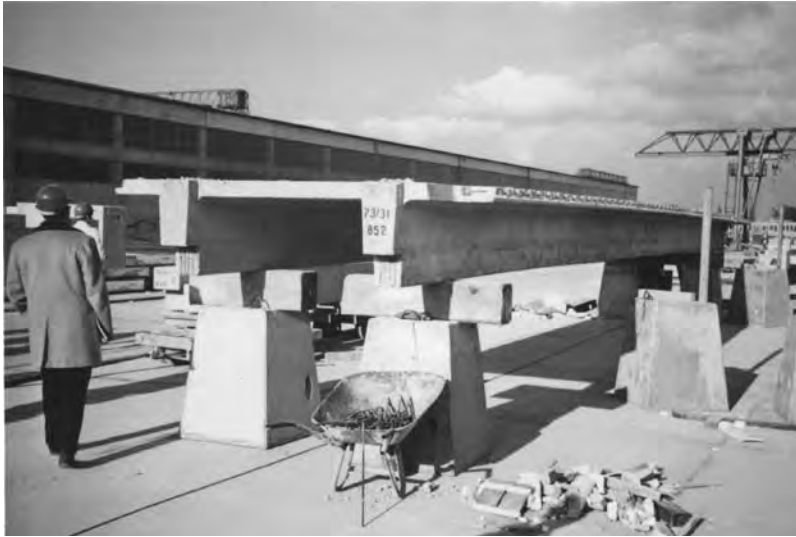
FIGURE 11.24 Double-tee precast, pretensioned concrete slab. (From Gerwick, B.C., Jr., Construction of Prestressed Concrete Structures , John Wiley & Sons, New York, 1996. With permission.)
