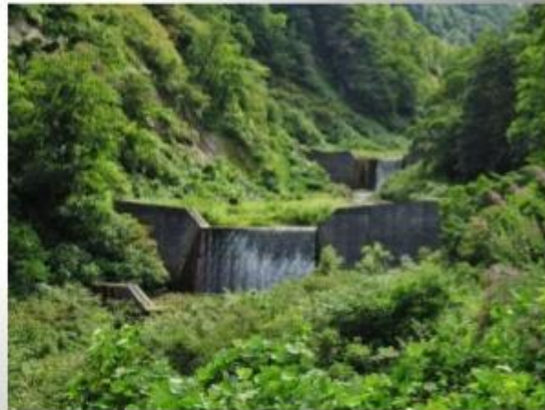
Fig. – A concrete check dam
