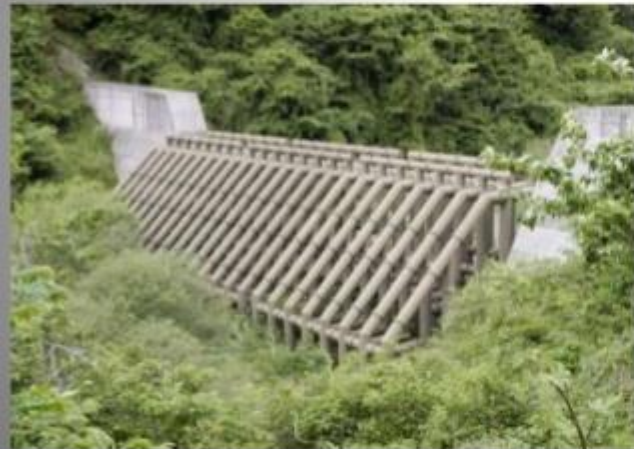
Fig. – A steel check dam
