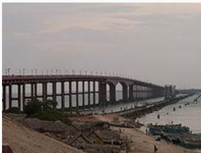
Pamban road (left) and rail (right) bridges, connecting the Indian mainland with the Pamban Island
