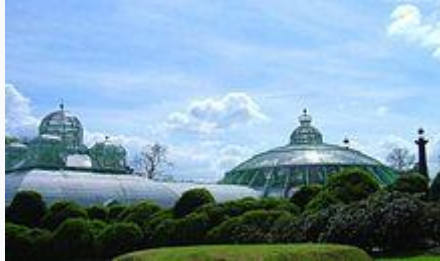
The Royal Greenhouses of Laeken, Brussels, Belgium . An example of 19th-century greenhouse architecture
